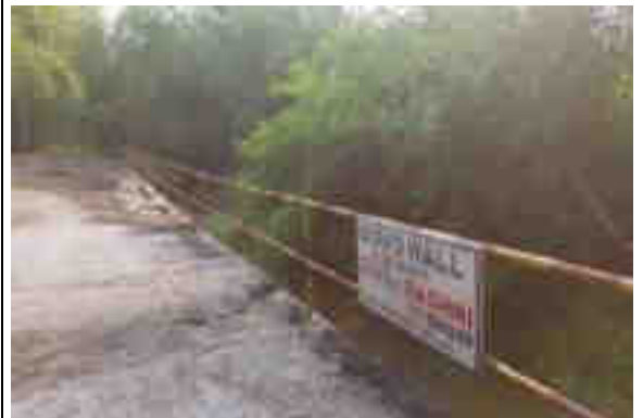
Construction of Guard Wall, Basantapur
