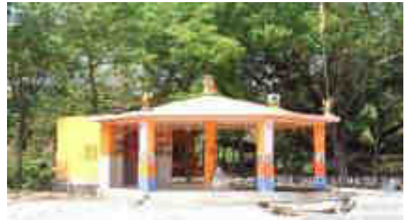
Construction of Community Prayer Centre (Mandir)
