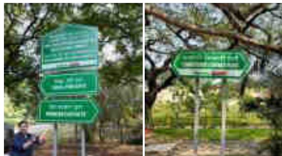
Installation of Signage's
