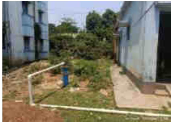
Construction of Water Drinking Facility, Kharagpur
