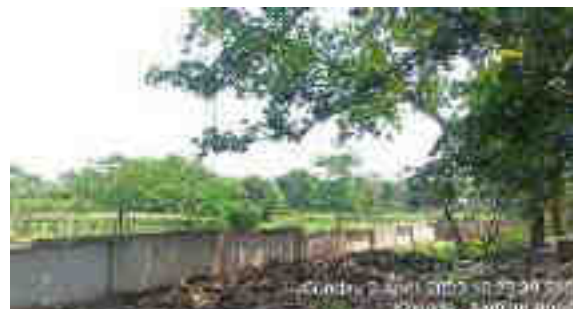
Construction of Boundary Wall of Community Prayer Centre (Mandir),
