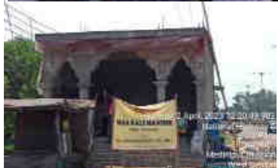
Construction of Community Prayer Centre (Mandir)
