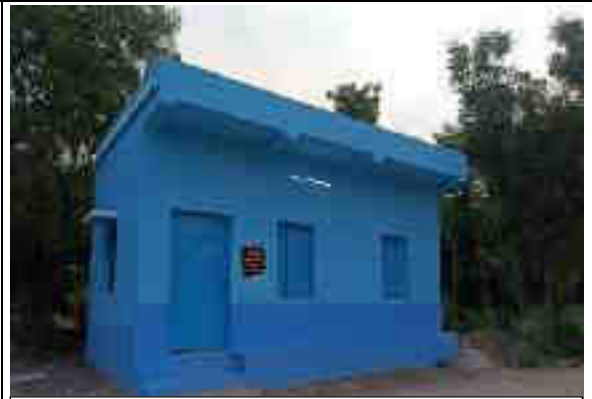
Construction of Community Centre Mahespur
